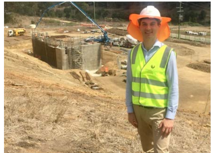
Queensland Urban Utilities' Project Manager, Jonathan Farrell, overseeing construction at the Lowood STP site (October 2018).
