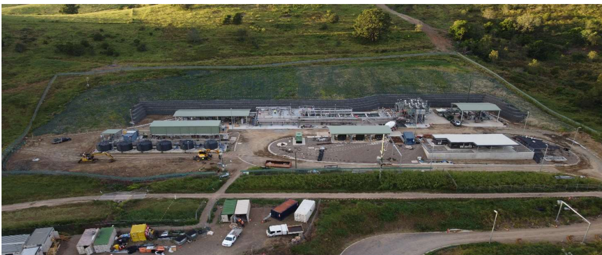
Image – Aerial view of Lowood STP (April 2021).
