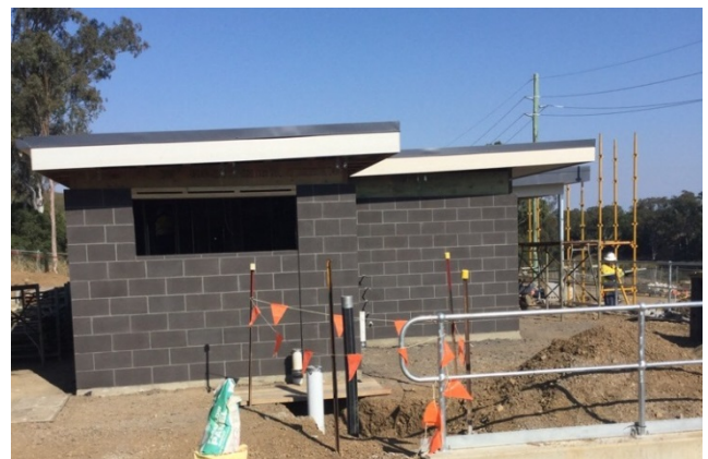
Above: Administration building under construction (Aug 2019)
