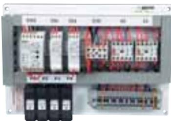
Relay/timer logic panel type controller Cat. No. TLP1
