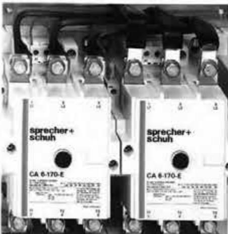
*Extremely low pick-up and hold-in coil consumption, compared with conventional contactors.*
