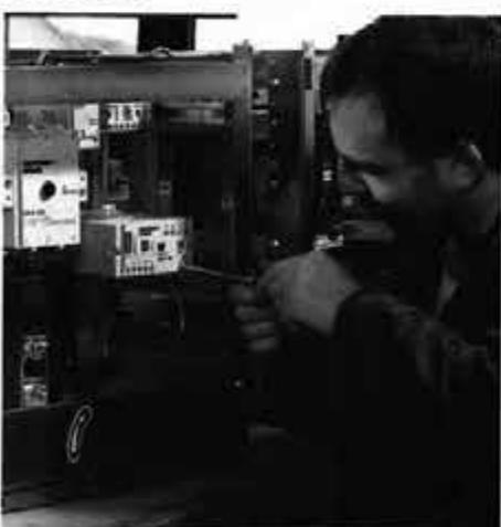
*Only 2 sets of flexible flat conductors are needed to wire all contactors up to 90kW, which makes wiring up starters a quick and simple job. Matching terminal lugs enable CEF 1 Electronic Motor Protection Relays to be mounted directly onto the contactors.*
