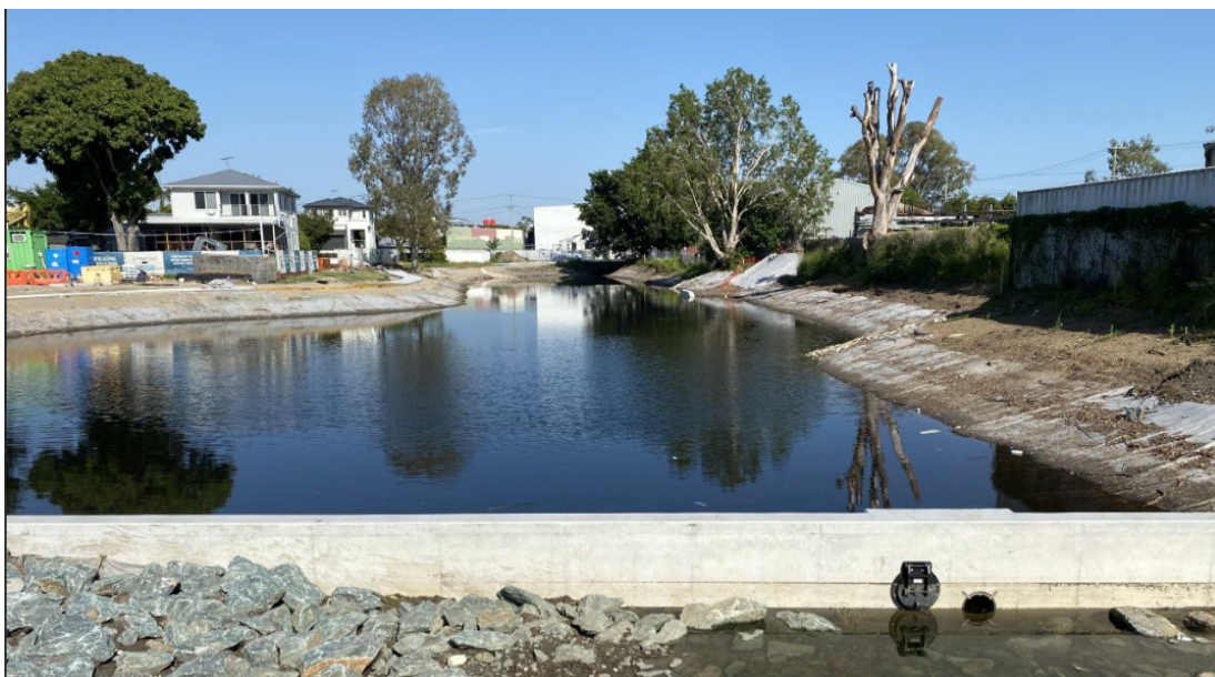
Image 3: Sediment basin one weir wall
