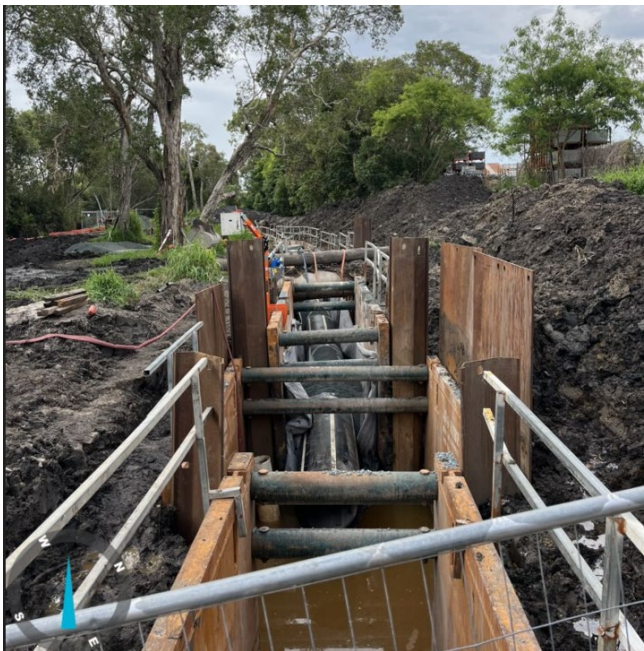
Image 8: Shore box excavation for the rising main pipe
