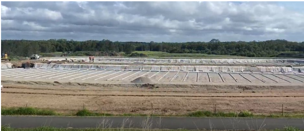
Image 10: Pipes placed on sand bed for the Southern Cross bio-retention basin
