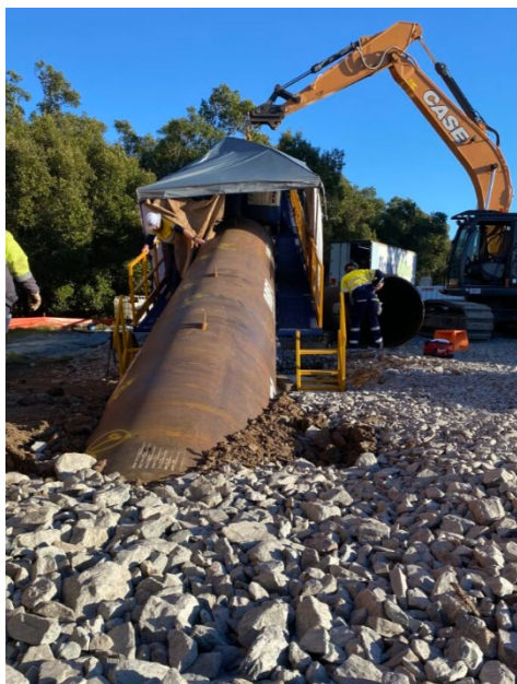
Image 6: Steel encasement under Nudgee Road
