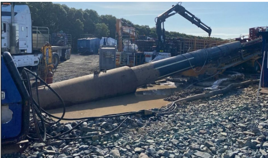
Image 7: Horizontal directional installing the rising main pipe
