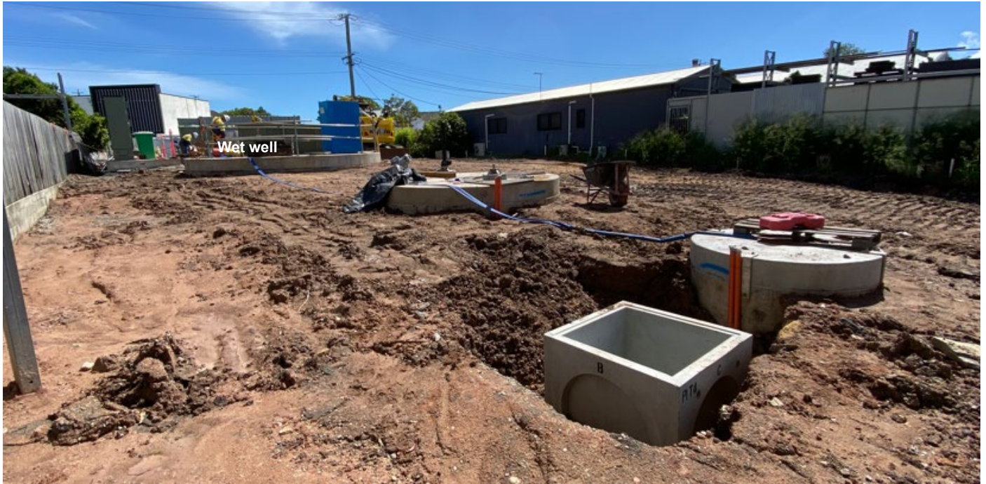
Image 4: Wet weather pump station
