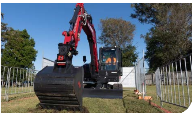
Breaking ground on the Cannery Creek project.
